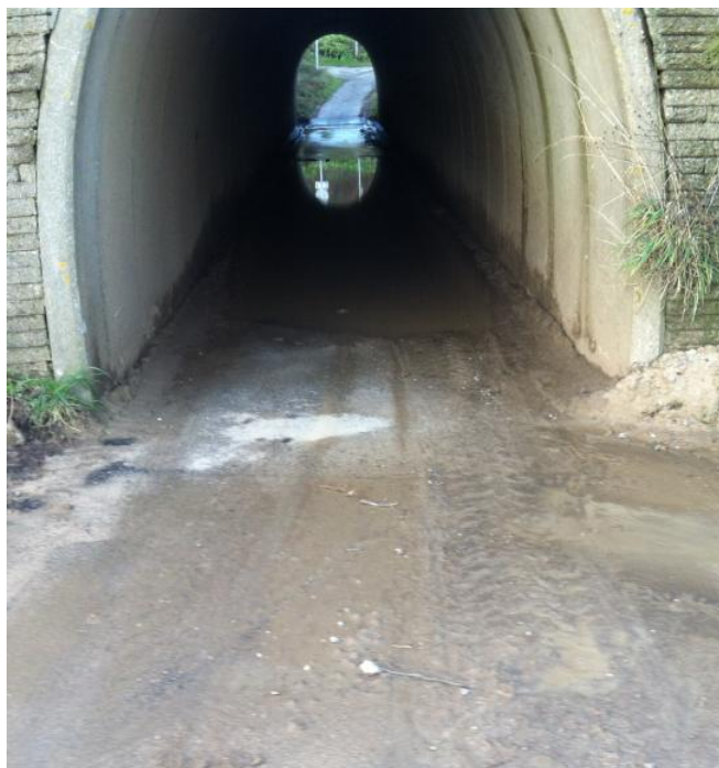
Tunnel of ... smat
